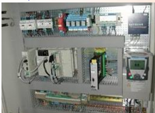
Control cabinet with embedded web server and proportional card
