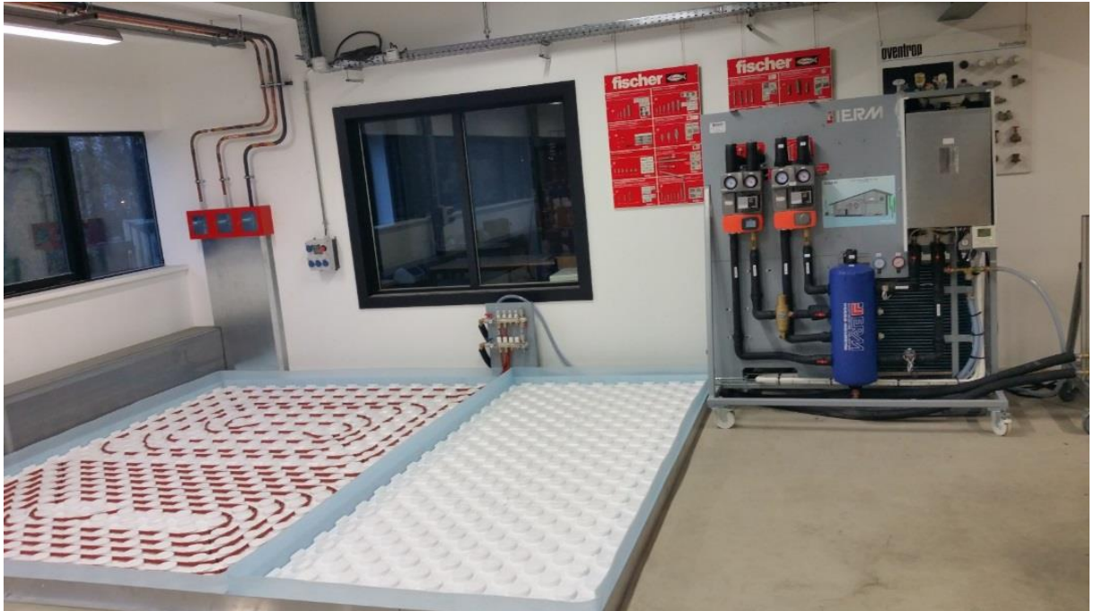
Example of a hydraulic underfloor heating system (PV20) with a 6kW reversible inverter air/water heat pump (PC60)
